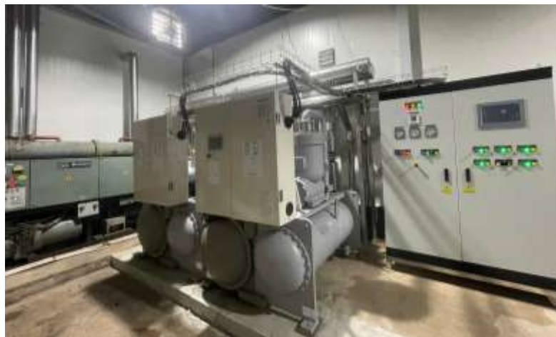
Figure 1. 1 Installation of Glycol Chiller system at Nafoods Tay Nguyen JSC
