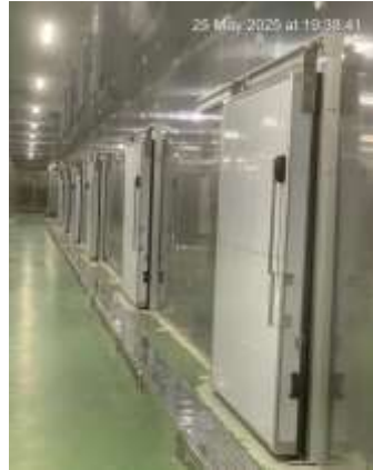
Figure 1. 2 Installing frozen booths and refrigeration system at Acecook project
