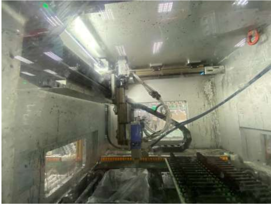
Figure 1.32 Three-axis Robot and vacuum chamber
