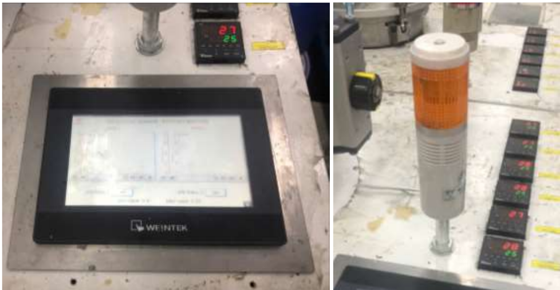
Figure 3.23 Installation of the HMI Screen, Warning Light
