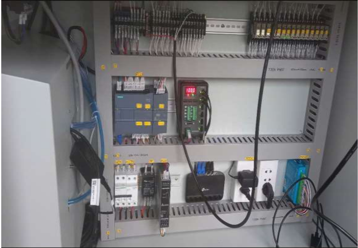
Figure 4.3. Electrical wiring and setup of the machine
