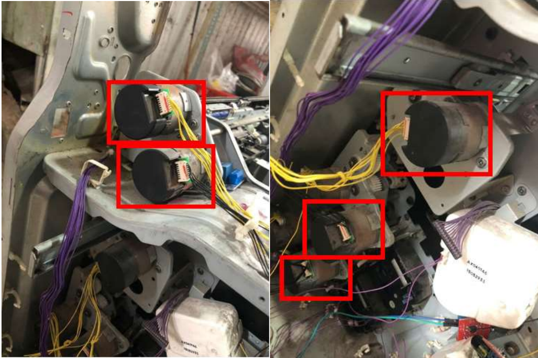
Figure 3.14 Actual installation positions of the motor
