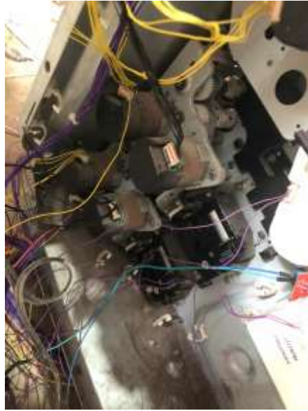
Figure 3.18 Actual installation position of the motor
