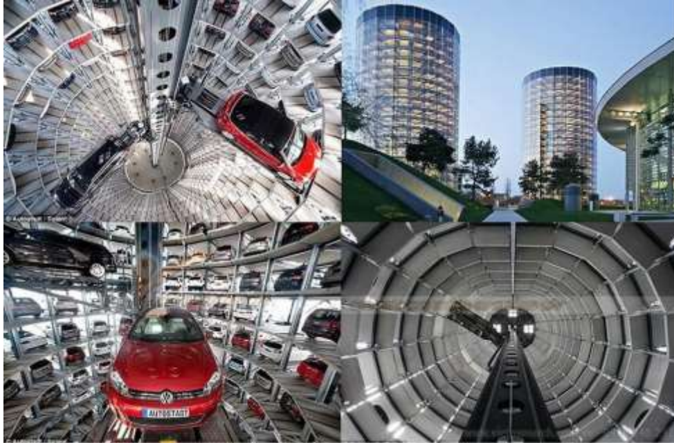
Figure 3.3 Multi-level Parking System Combined with Lifting Mechanism
