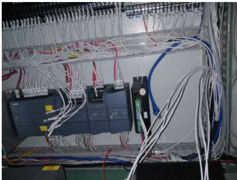
Figure 6.4 Electrical Cabinet Under Installation
