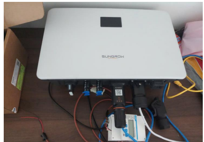
Figure 17: The inverter needs to be connected to PPC(SMA, Sungrow, DEYE)
